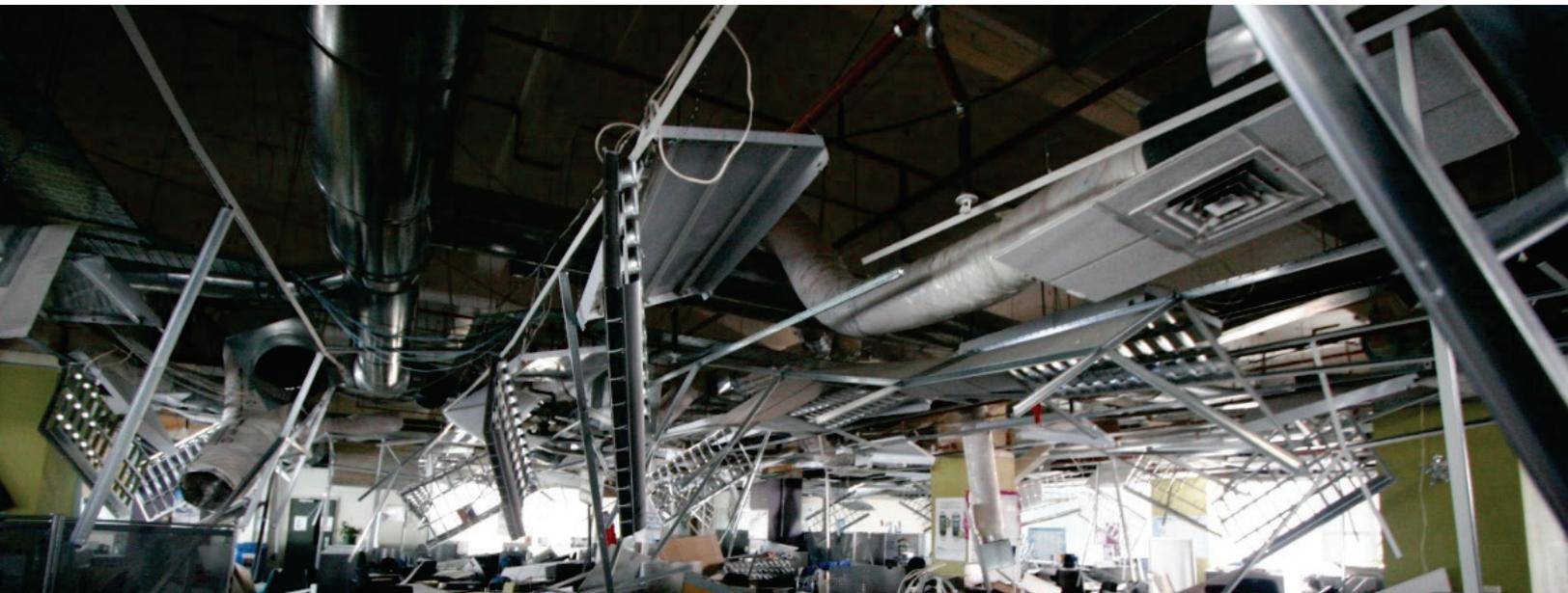
Interior damage in this Christchurch, New Zealand office building after the 2011 earthquake demonstrates the safety concerns and length of time it might take to restore nonstructural elements of a building to usable condition.
