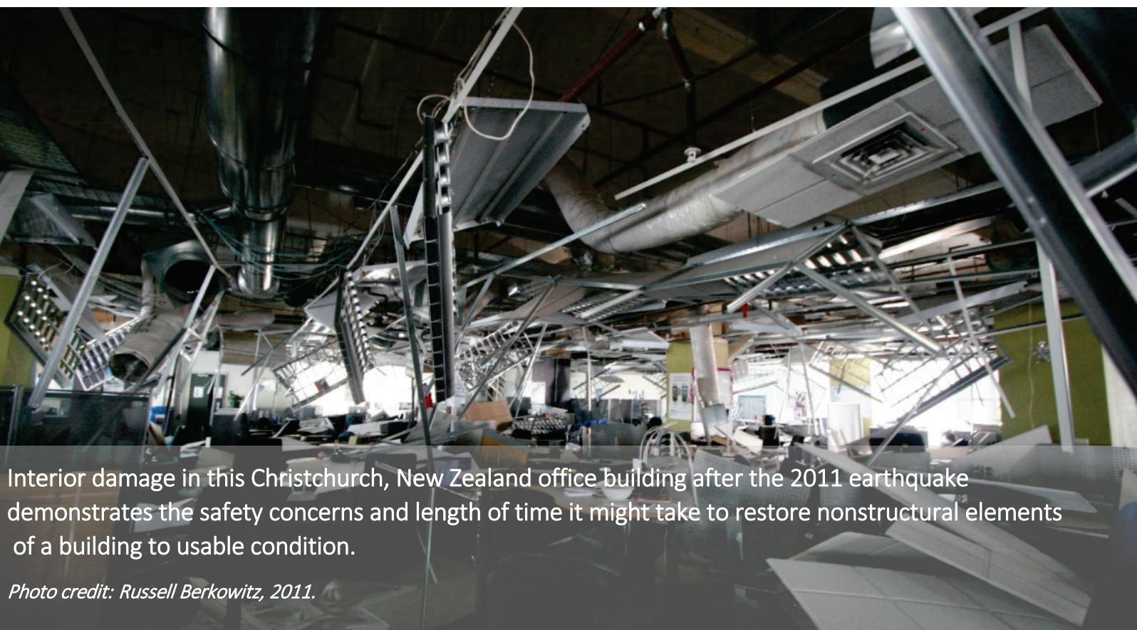
Interior damage in this Christchurch, New Zealand office building after the 2011 earthquake demonstrates the safety concerns and length of time it might take to restore nonstructural elements of a building to usable condition.
